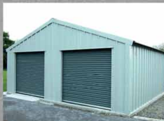
9.1m x 7.3m Double Garage Unit
