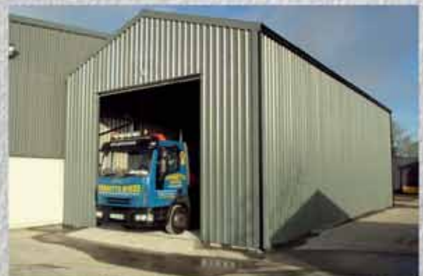
15.2m x 7.3m High Storage Unit
