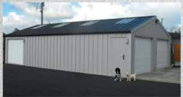
12.2m x 7.3m Double Garage Unit
