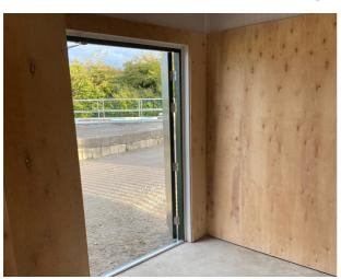
At Shanette, we offer the option to finish the interior walls of your unit with fire-rated 18mm plywood sheets. This allows you to easily mount components, panels, cable trays, and more.
