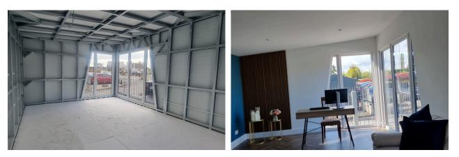
Shanette can provide 600mm steel centres, ensuring an easy and hassle-free installation for slabbing internal roofs and walls in our units. Additionally, our frames can be pre-drilled to accommodate your electrician's needs as per the image below.
